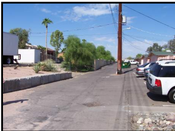
Break in wall for incoming channel flow
