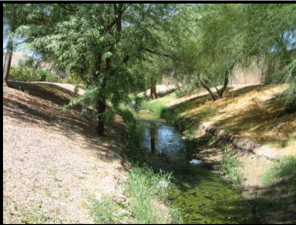
Channel behind Belle Rive apartments
