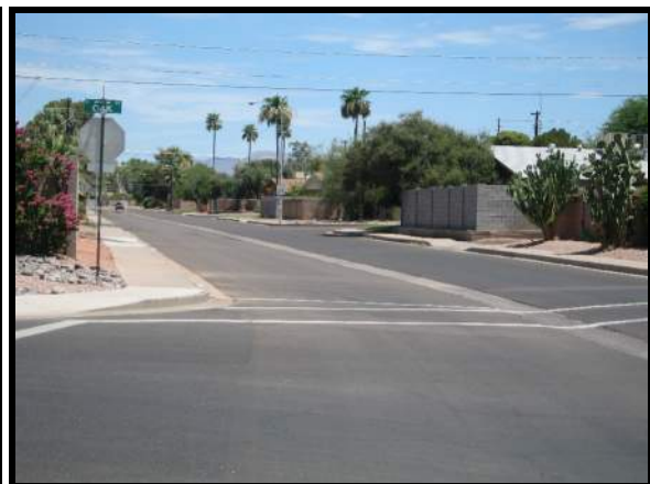
87 th St inverted crown section
