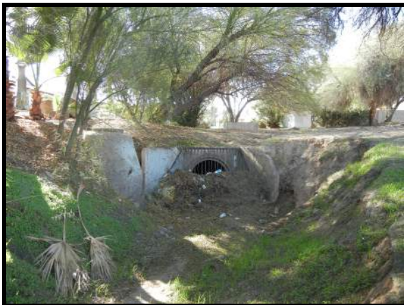
Storm drain entrance at 84 th PI
